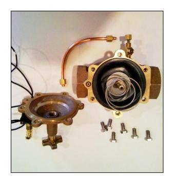
**3.** Remove diaphragm spring and diaphragm assembly from valve body.
