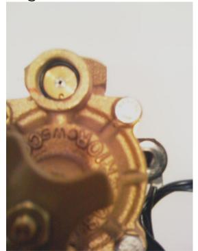
1. Remove solenoid retainer nut and slide solenoid coil and Uframe off of solenoid post
