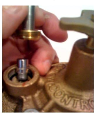
Solenoid cavity: The center port is the exhaust port. The other port connects the solenoid cavity to the diaphragm chamber
